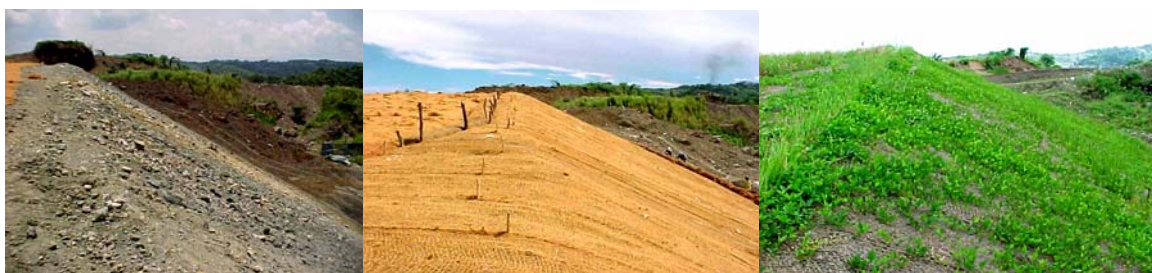
Figure 5: Rehabilitating the hillsides
